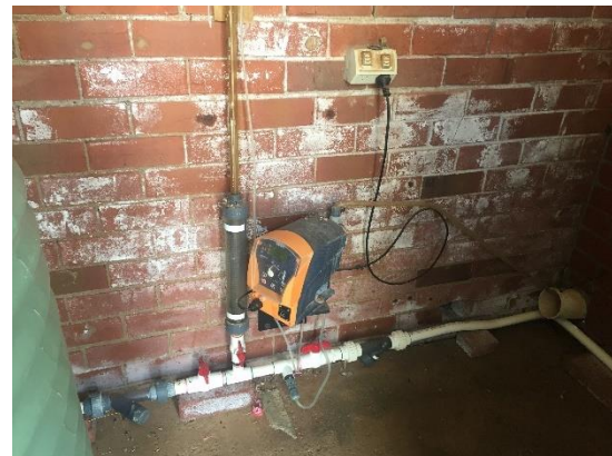
Figure 2-35 Dunedoo Chlorine dosing pump
