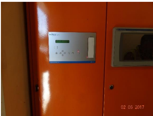
Figure 2-42 Mendooran HMI & FLYGT display
