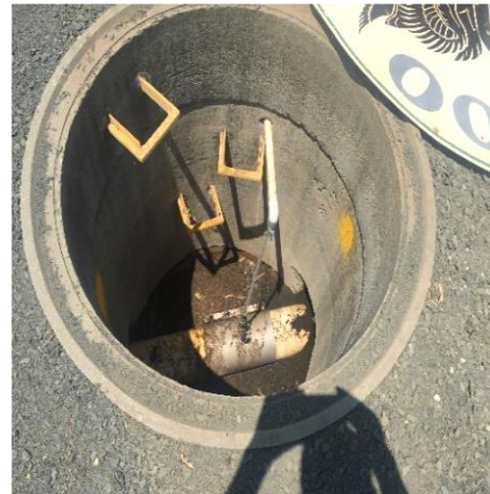
Figure 2-33 Dunedoo Chlorine dosing point
