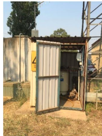
Figure 2-10 Bugaldie pump house
