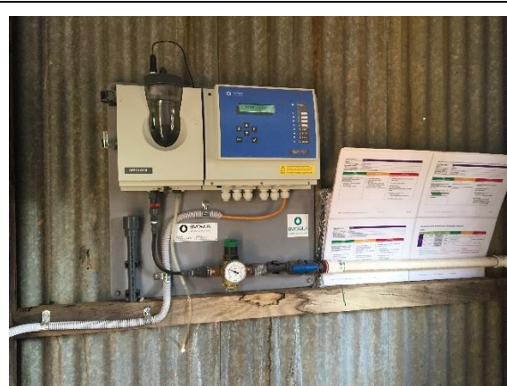
Figure 2-37 Kenebri Chlorine analyser
